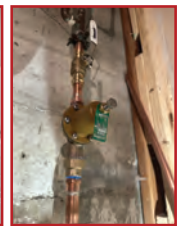
PRV INSTALLATION AND REPLACEMENTS
