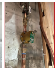
PRV INSTALLATION AND REPLACEMENTS
