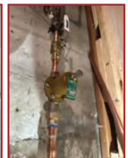
PRV INSTALLATION AND REPLACEMENTS
