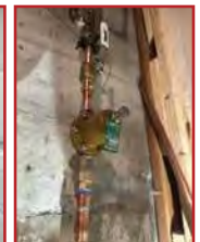
PRV INSTALLATION AND REPLACEMENTS
