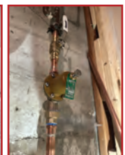
PRV INSTALLATION AND REPLACEMENTS
