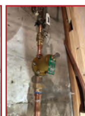
PRV INSTALLATION AND REPLACEMENTS
