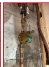
PRV INSTALLATION AND REPLACEMENTS
